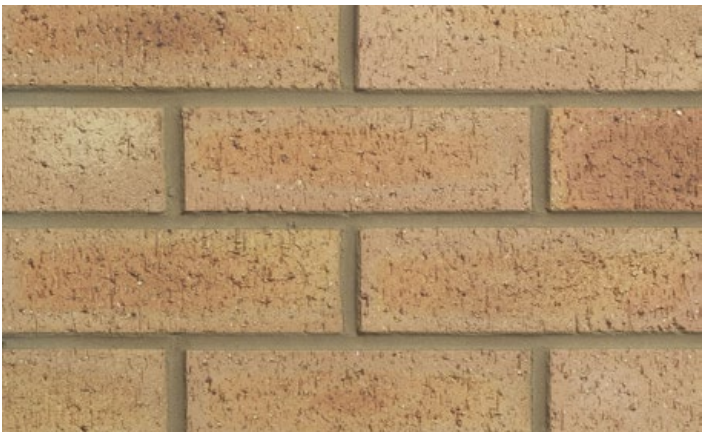
BRICK Standard brick veneer or bagged brick plaster finish (white wash) LOW CONTRAST MORTAR Reduce the contrast of mortar with the adjacent brick, by using a light mortar for lightly coloured bricks, and a darker mortar for dark bricks.
