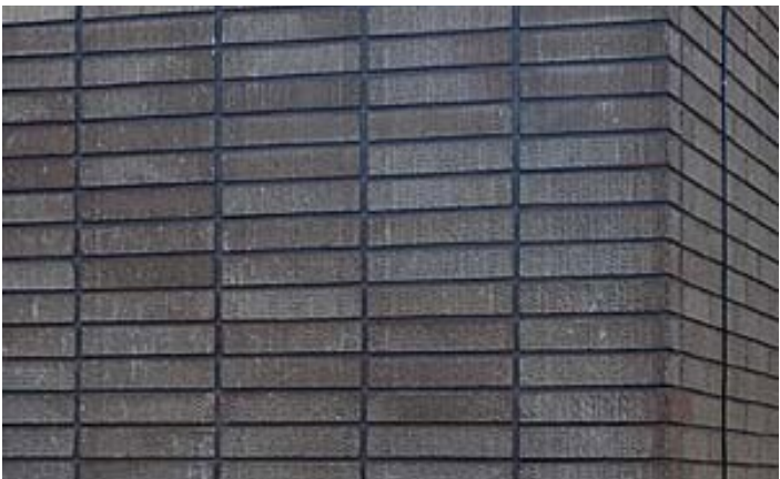
BRICK Standard brick veneer or bagged brick plaster finish (white wash). Stacked brick veneer acceptable. LOW CONTRAST MORTAR Reduce the contrast of mortar with the adjacent brick, by using a light mortar for lightly coloured bricks, and a darker mortar for dark bricks.
