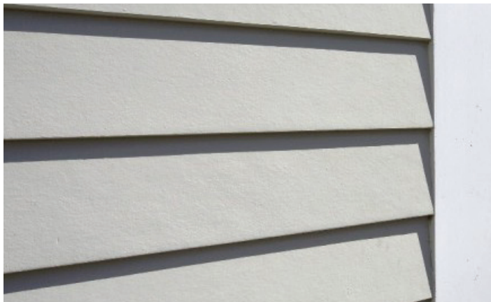
WEATHERBOARD Weatherboard cladding
