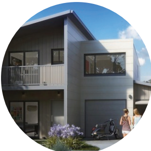
BROKEN DOWN FACADE / LAYERING TO HOME ENTRY
