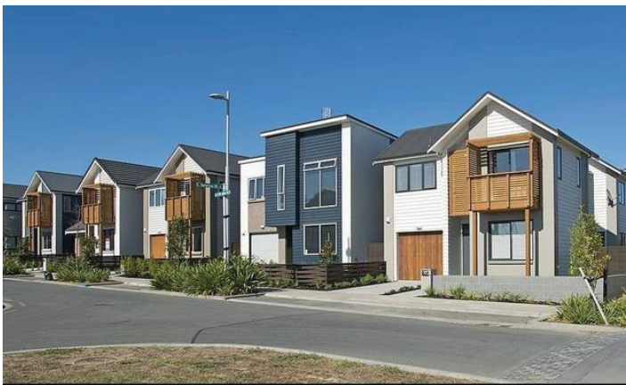
TIMBER CLADDING Stained, painted or natural. Vertical Shiplap or Horizontal bevel back weatherboard. Ensure any natural timber meets minimum H3.2 treated. All rough sawn pine to be stained or painted.
