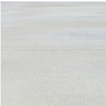
CONCRETE SEALER On Concrete Flooring
